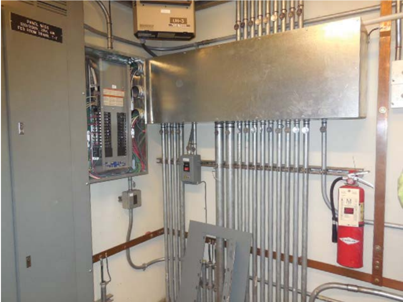
King Street North Photo #4 – Shared Trough for AFC Panel NF, Source Panel NESS, and Panel NES
