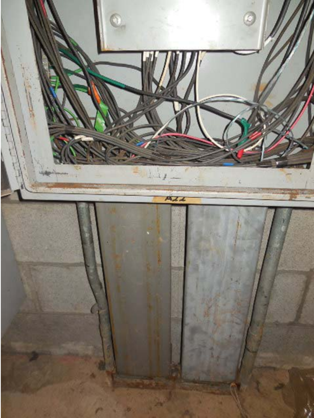
Mt. Vernon Photo #3 – AFC Panel (F) Walker Duct to transition to Mezzanine Floor
