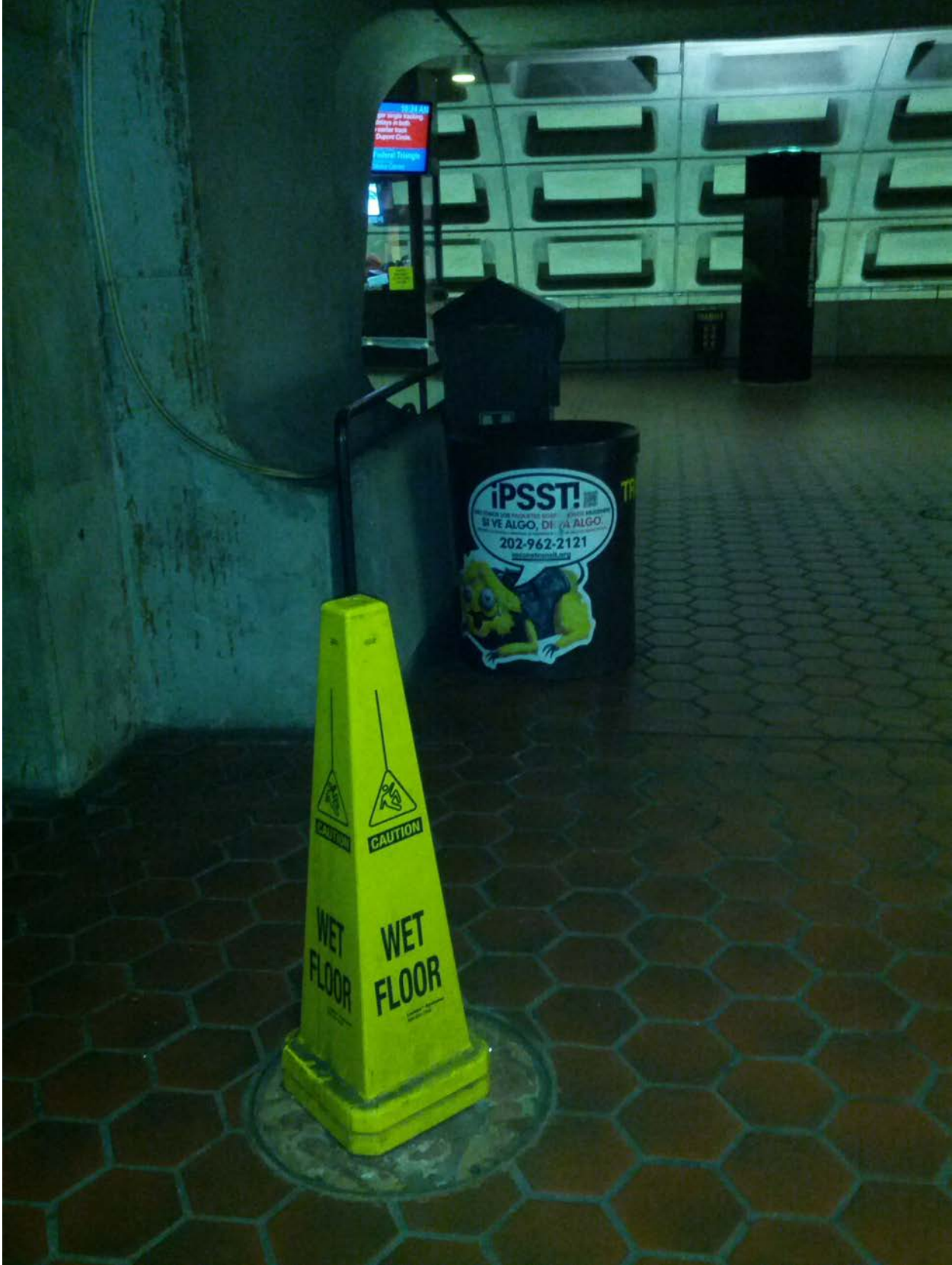
Photo #9: E02 Shaw-Howard U (South) – Mezzanine level handholes
