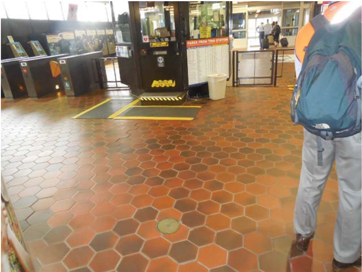
Photo #1: C10 Reagan Airport South – Handholes at Mezzanine & Kiosk
