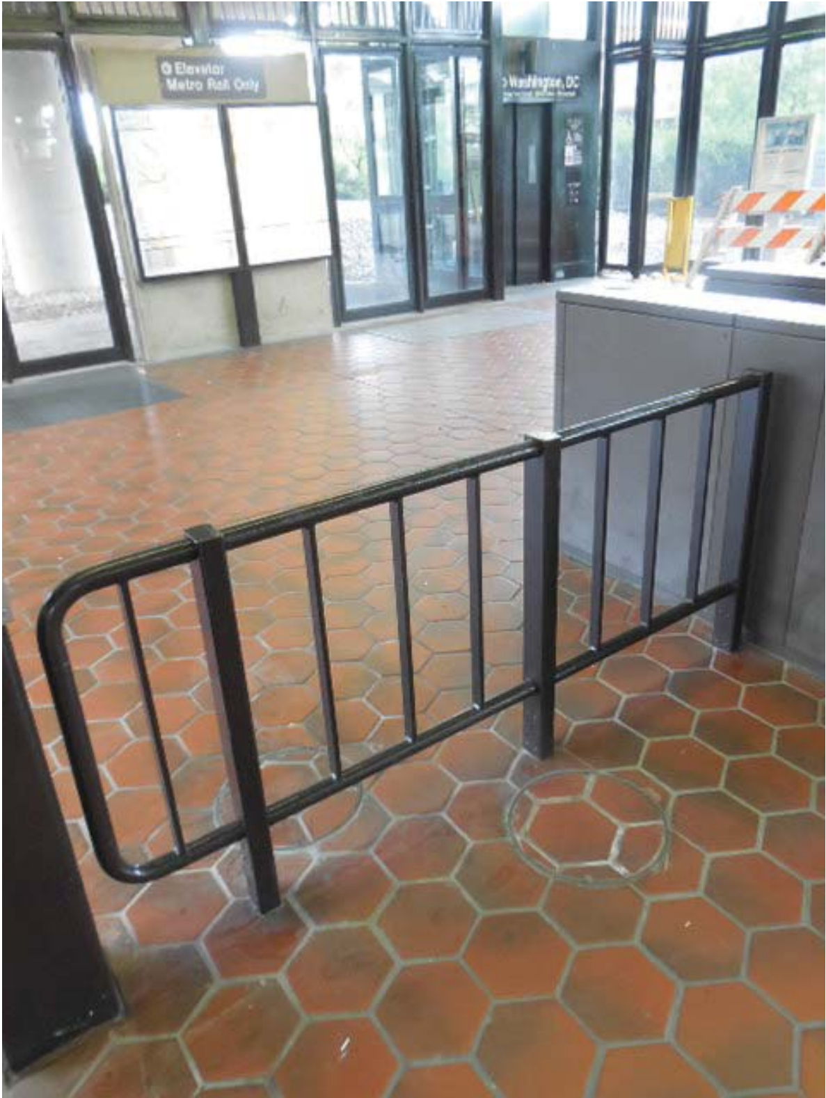
Picture 5: C10 Reagan Airport North – Handholes at Mini-Mezzanine
