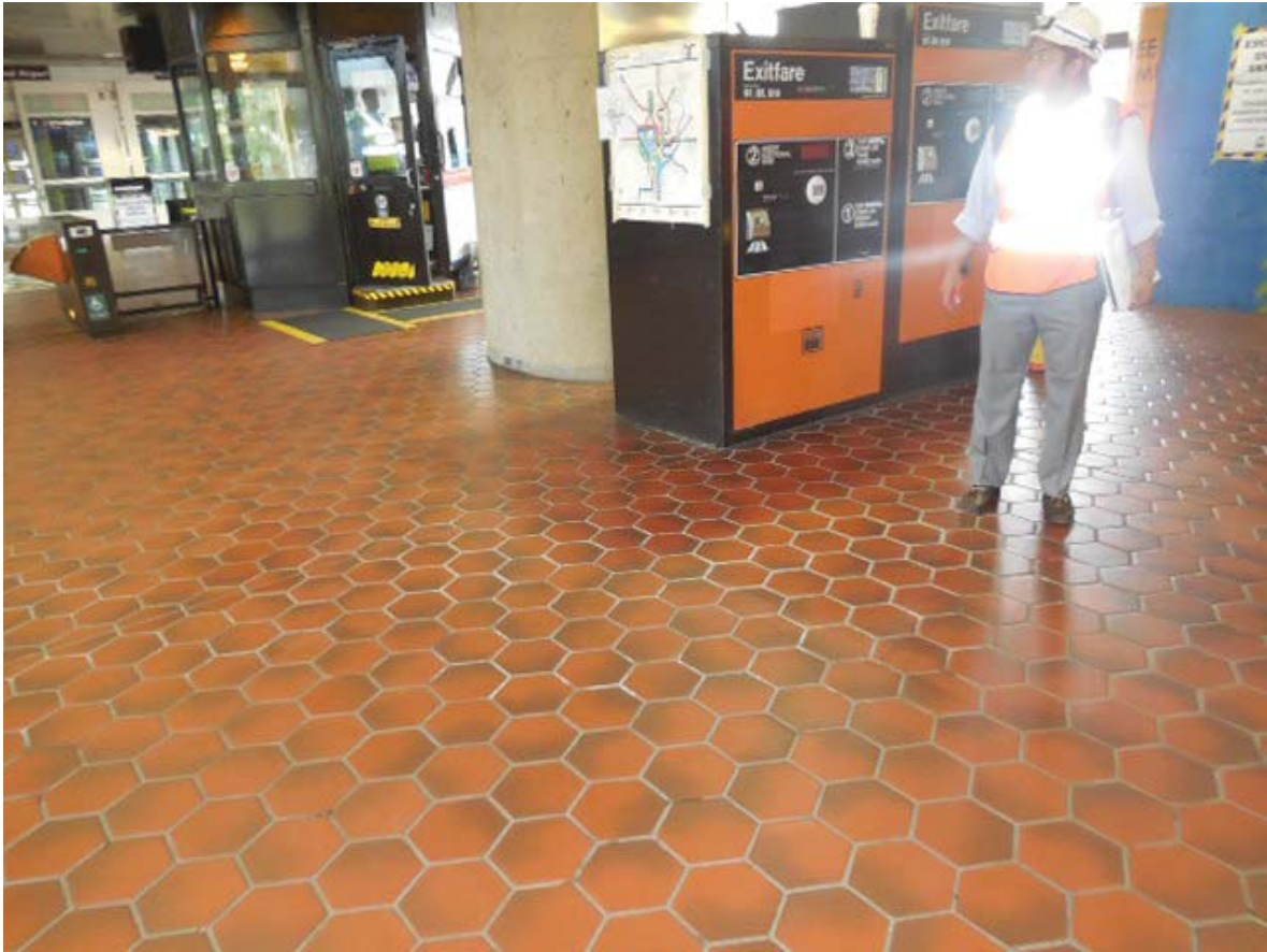
Picture 1: C10 Reagan Airport North – Handhole at Mezzanine
