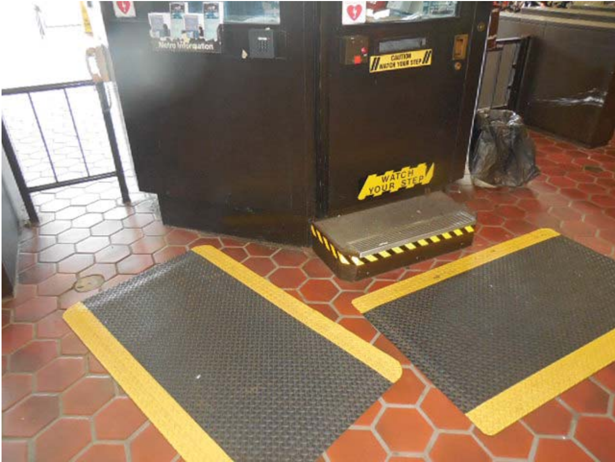
Photo #1: C15 Huntington North – Handholes at Mezzanine
