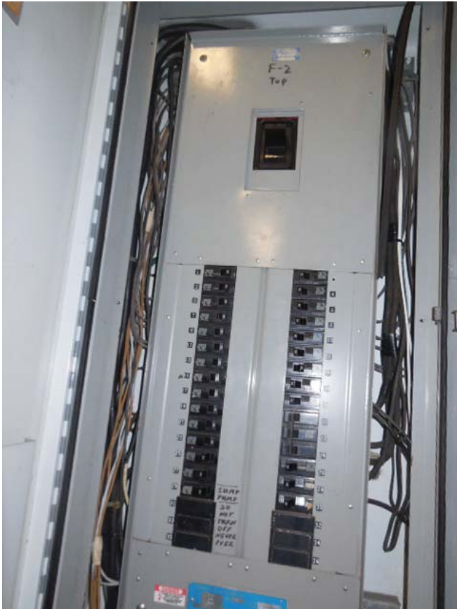
Photo #12: C13 King Street (South) – Panel F2 in Room C103
