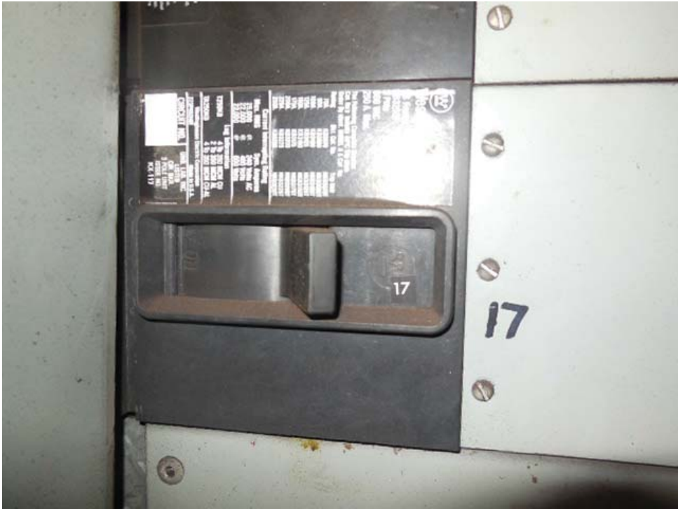
Photo #9: C09 Crystal City – Source breaker for AFC Panel 2MM on Panel M
