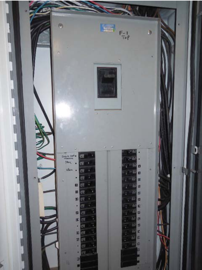
Photo #10: C13 King Street (South) – Panel F1 in Room C103
