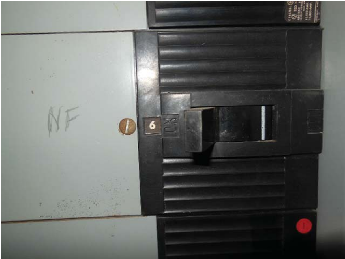
Photo #7: C15 Huntington North – Panel NPOE – Circuit #6 to de-energize AFC Panel NF
