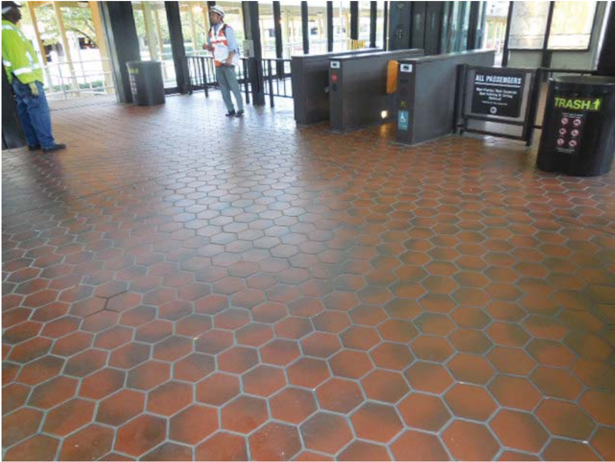
Picture 2: C10 Reagan Airport North – Handholes at Mini-Mezzanine
