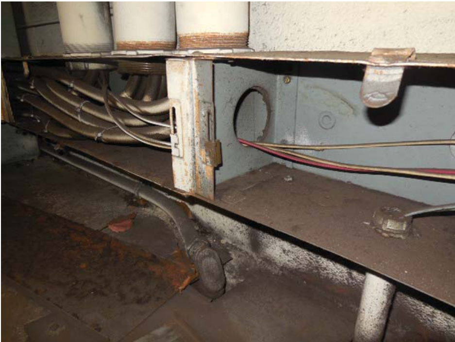
Photo #4: C09 Crystal City – Other panels feeding into common trough in Room C302
