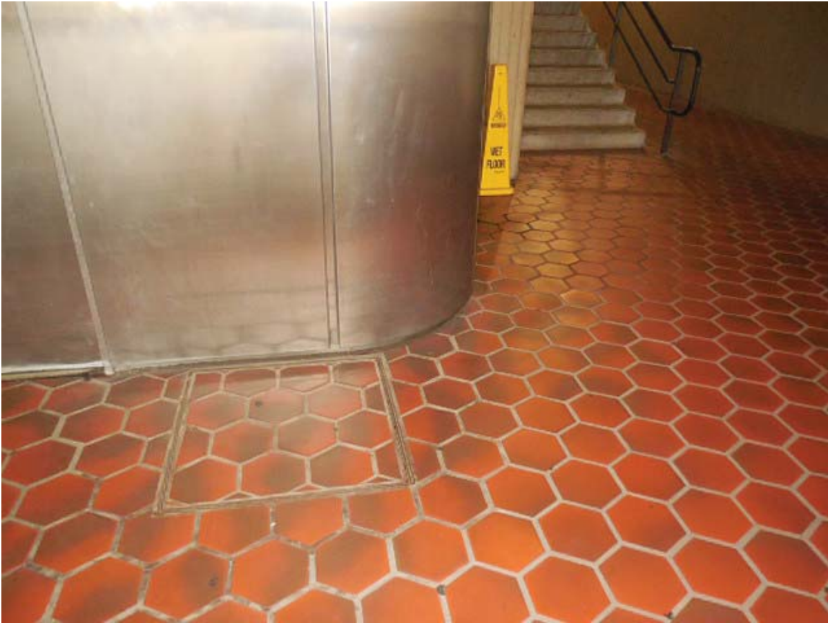
Photo #2: C15 Huntington North – Handholes at Mezzanine
