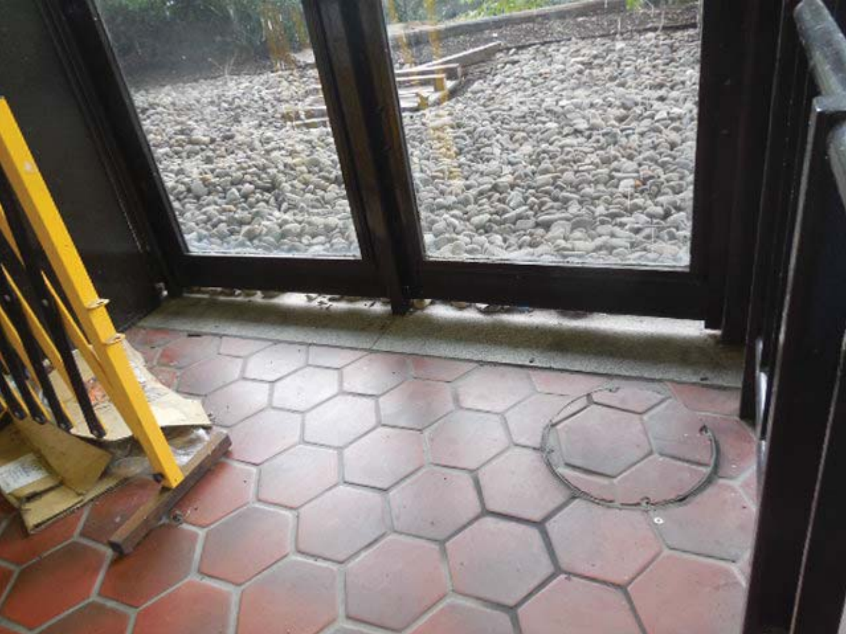
Picture 6: C10 Reagan Airport North – Handholes at Mini-Mezzanine
