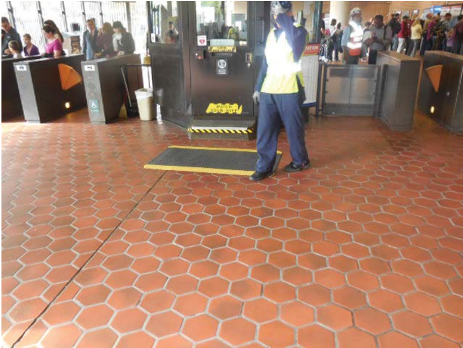
Photo #1: C13 King Street (South) – Kiosk at mezzanine level
