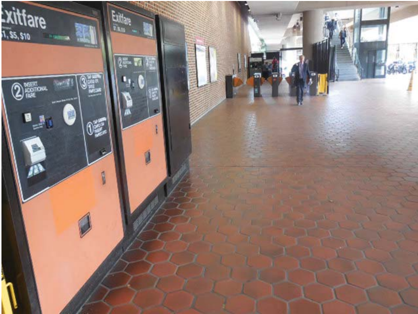
Photo #5: C13 King Street (South) – Mini-mezzanine mezzanine area
